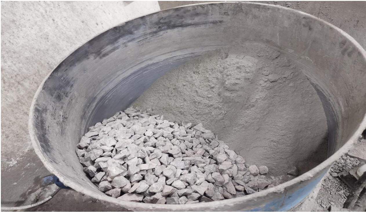
Fig.9: Dried concrete mixture before addition of water and super-plasticiser
