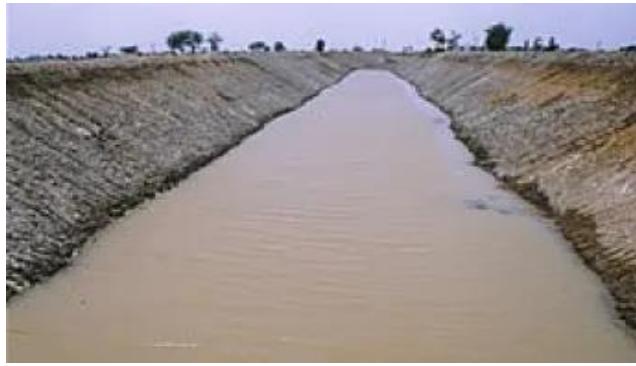
Fig 4.2.6 Boulder Lining
