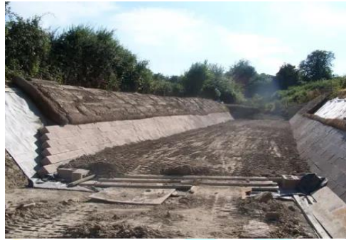
Fig 4.2.2 Brick Lining
