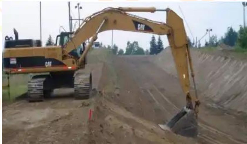
Fig 4.2.4 Compacted Earth Lining
