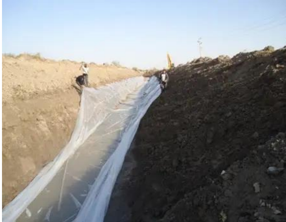
Fig 4.2.5 Plastic Lining
