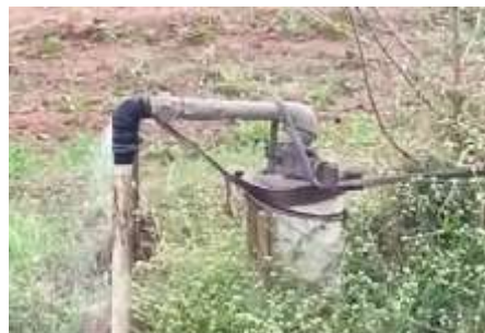
Figure 7: Testing of submersible motor at farm
