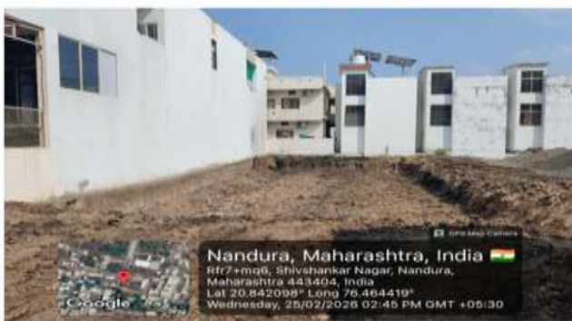
Fig. 1: Proposed site for excavation adjacent to existing building
