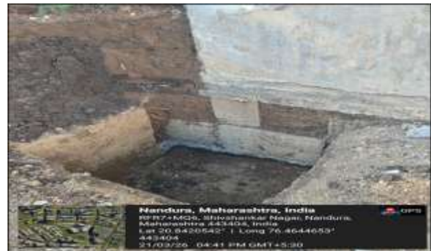
Fig. 2: Exposed Eccentric Footing of Existing Building
