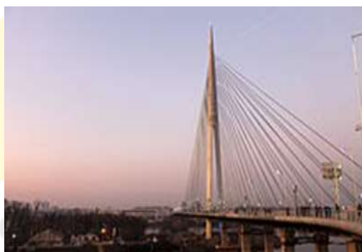
Fig.1 Cable stayed Bridge
