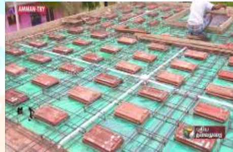
Fig 4.5 Filler material used .
