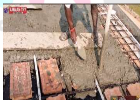
Fig 4.15 Filler material used
