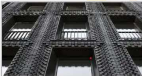
Fig 4.30 Interlocking brick used for exterior.
