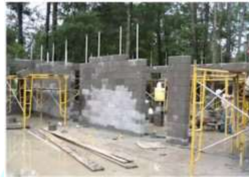
Fig 4.26 Dry stacking the wall
