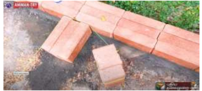
Fig 5.10STEP 4: Begin Laying Interlocking Bricks:
